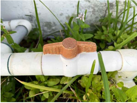
Main Water Shut Off
