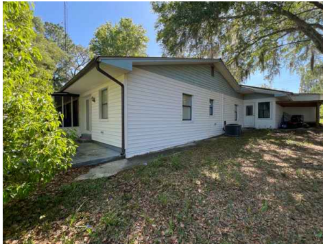
Left Rear Corner
