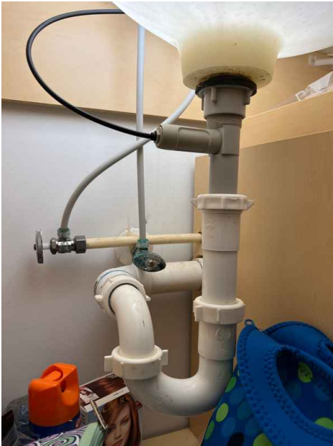
Bathroom 1 Sink Right
