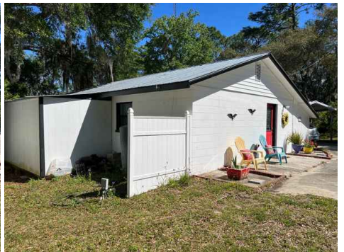
Front Left Corner
